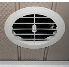
EZ Soffit Vent installed
